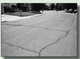
volume facilities such as Interstate and primary highways, fatigue is best countered using a total HMA thickness that keeps the bending strain under the vast majority of heavy traffic loads below a threshold of about 70 microstrain. This will ensure that cracks do not originate at the bottom of the structure and propagate up to the surface. Thus, the need for full-depth patching or complete reconstruction of the HMA can be avoided.
