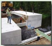
The mid-section of the precast superstructures for a bridge on *M*-115 is placed as part of the Michigan DOT's performance contracting project.
