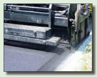
The asphalt paving technique called the Safety Edge is gaining momentum across the country as State transportation departments strive to protect motorists from run-off-the-road crashes. The Federal Highway Administration recommends that States use the safety edge technique—particularly on two-lane roads with unpaved shoulders.
